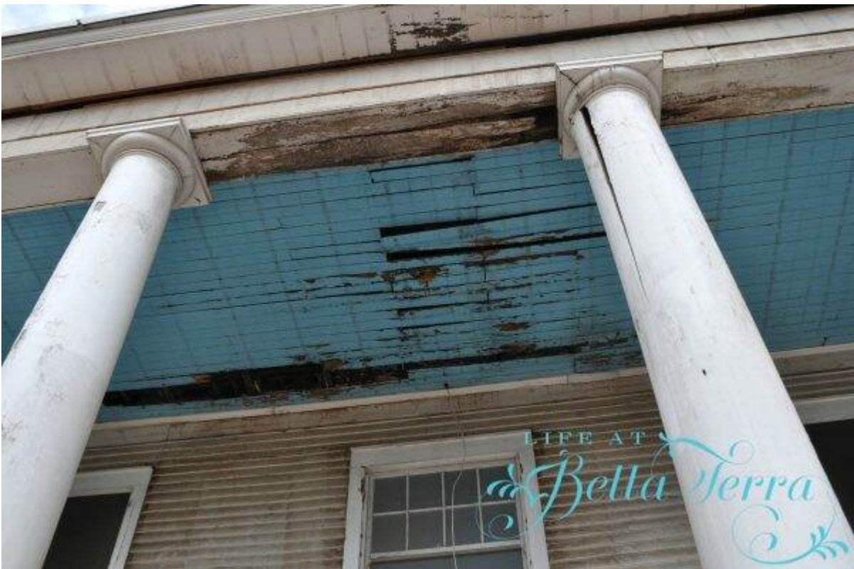
When we removed the aluminum siding from the underside of the porch ceiling, we found a great deal of water damage.
